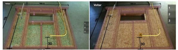
Figure 13 - Superimposition of the virtual model over the real one showing positioning flaws
