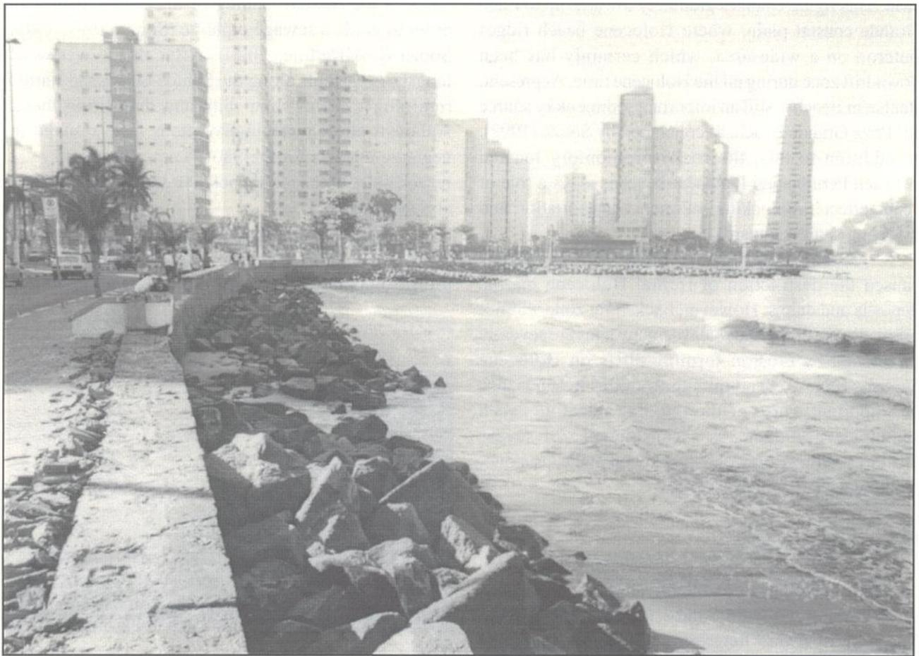
Figure 5 - Severe erosion on São Vicente Beach (central sector). Stone-groins and -revetment and concrete-wall are not able to protect the beach against erosion. Porchat Island, that was artificially connected to the continent, is at the upper-right side of the photo.
