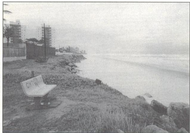
Figure 4 - Severe erosion on Itanhaém Beach (central sector). Note that the embankment and the stone-revetment placed there in order to protect the beach against erosion are being destroyed.
