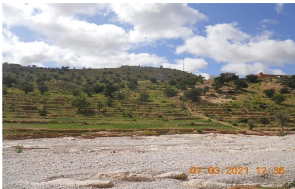
Picture1: The Aouerga's main channel at its lowest point following the drainage of floodwaters.
