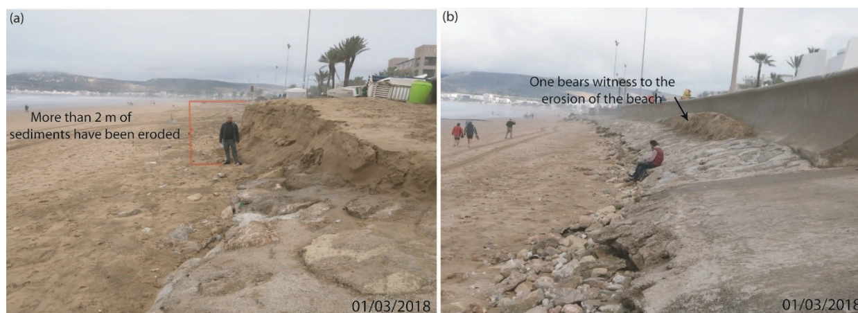
Figure 9. Significant erosion was observed in the central and southern sectors of Agadir Beach following the storm on March 1, 2018. Photos (a) and (b) show a large quantity of sand carried offshore by waves exceeding 5 meters, leaving behind a micro-cliff several meters high (a) and clear signs of marine erosion (b). (Source: personal photographs).
