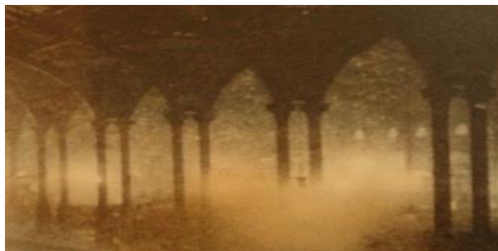
Figura 15 - Liverpool Street Station
