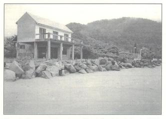
Figure 2 - Severe coastal erosion on Guaraú Beach (central sector). This site is northward from the stone-groin placed at Guaraú River mouth.
