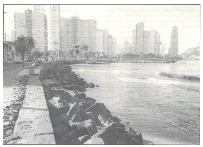
Figure 5 - Severe erosion on São Vicente Beach (central sector). Stone-groins and -revetment and concrete-wall are not able to protect the beach against erosion. Porchat Island, that was artificially connected to the continent, is at the upper-right side of the photo.
